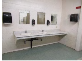
4 SJA Womens washroom - sink area
