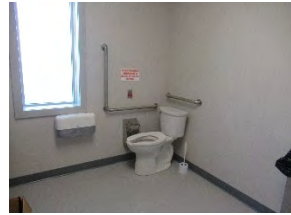
3 MFS Universal washroom toilet area
