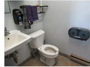
6 UWY Womens washroom toilet area
