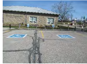
3 MCC Accessible parking
