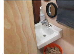
5 CCC Washroom toilet area 2
