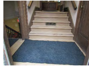
3 SJL - Stairs to main level
