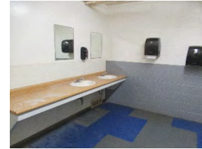
12 SJA Mens washroom sink area
