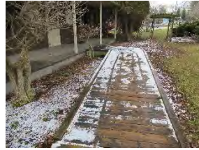
4 EYSO - Ramp to entrance
