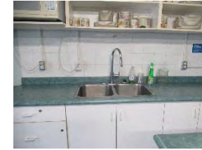
5 ELH Kitchen sink area
