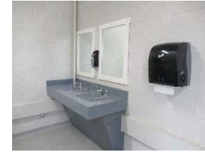
6 ELPW - Mens washroom sink area
