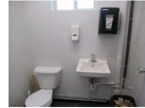
6 STJW - Mens washroom sink area
