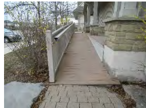
18 BCC Exterior ramp
