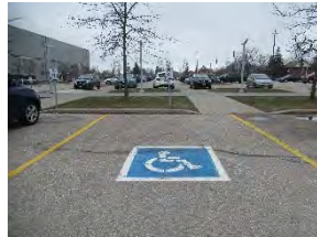
2 WMC - Accessible parking front
