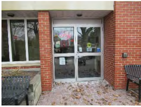
1 Elmira Library - entrance
