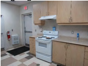
15 MCC Kitchen stove area
