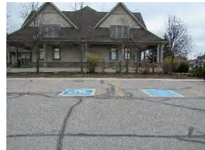
17 BCC Accessible Parking
