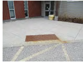
3 BFS - tactile warning plates 2
