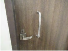
15 BFS Mens Changeroom washroom door
