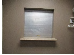
4 MCC Serving counter
