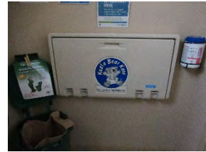
10 SJL - lower level washroom change table
