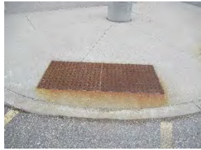
2 BFS - tactile warning plates
