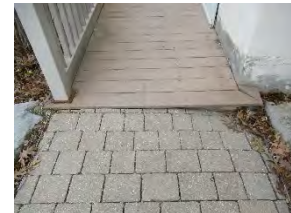
19 BCC Exterior ramp - lip
