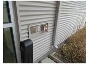
4 BFS - entrance controls
