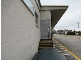
1 St Jacobs Warehouse - Entrance
