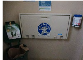
10 SJL - lower level washroom change table
