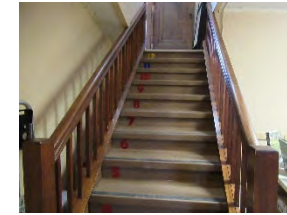
6 SJL - stairs to lower level
