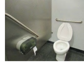
13 MCC Womens washroom stall
