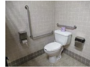
13 FFS - Womens washroom stall
