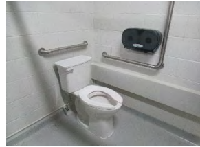
3 ELPW - Womens washroom toilet stall
