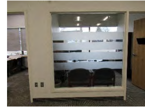
12 WAO office area window glazing
