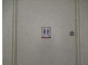
18 WAO Basement - unisex washroom
