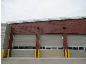
1 Breslau Fire Station
