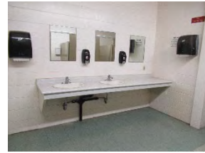
4 SJA Womens washroom - sink area
