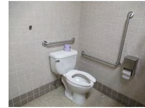
6 FFS - Mens washroom stall toilet area
