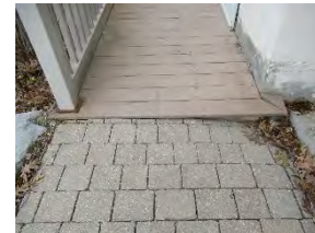
19 BCC Exterior ramp - lip
