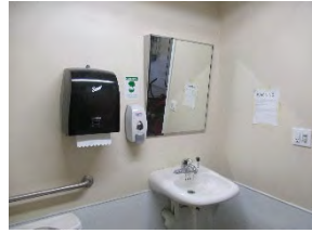
4 BS - Individual washroom sink area
