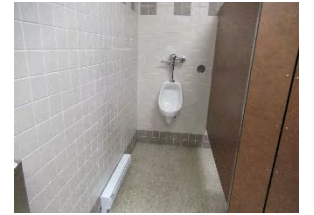
7 FFS- Men's washroom urinal area
