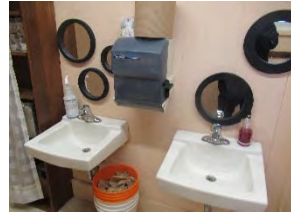
3 CCC Washroom sink area
