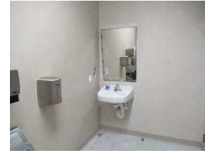
5 HCC washroom sink area
