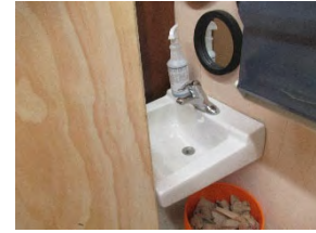
5 CCC Washroom toilet area 2
