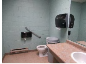
2 BLCC - Individual Washroom toilet area
