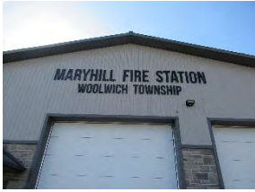
1 Maryhill Fire Station
