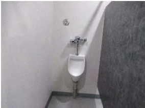
8 MFS Mens Changeroom urinal
