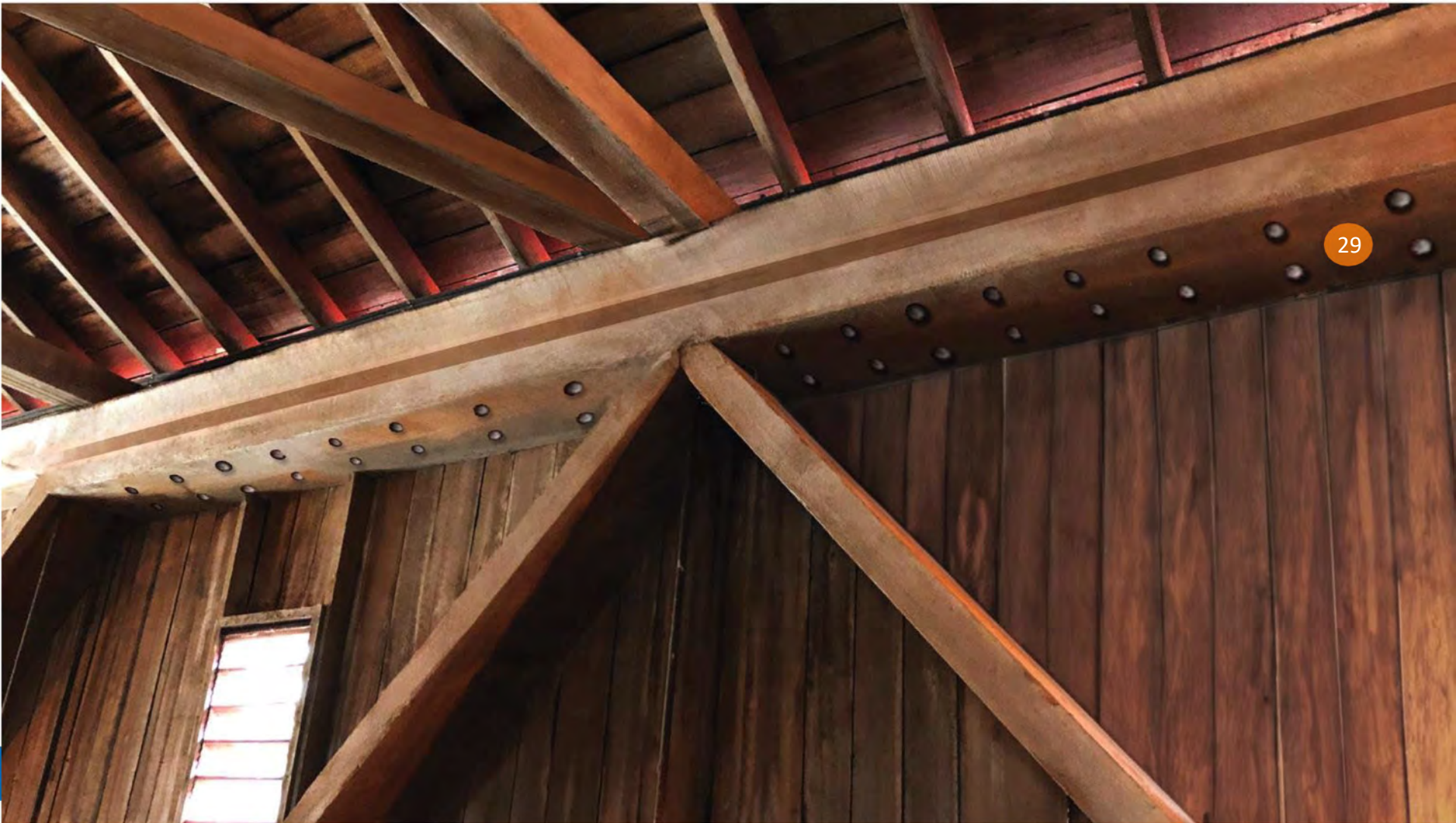
29 Reinforce top chord with lower top chord
