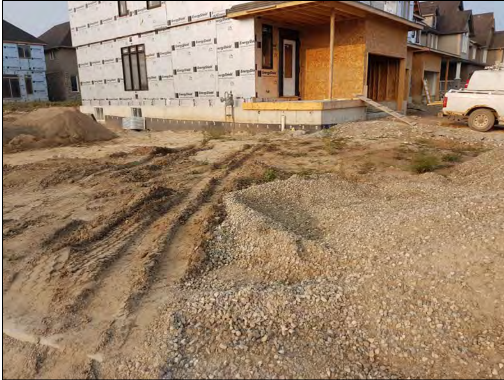
Photo 3. "Typical" Soil Conditions for Street Trees in New Subdivisions
