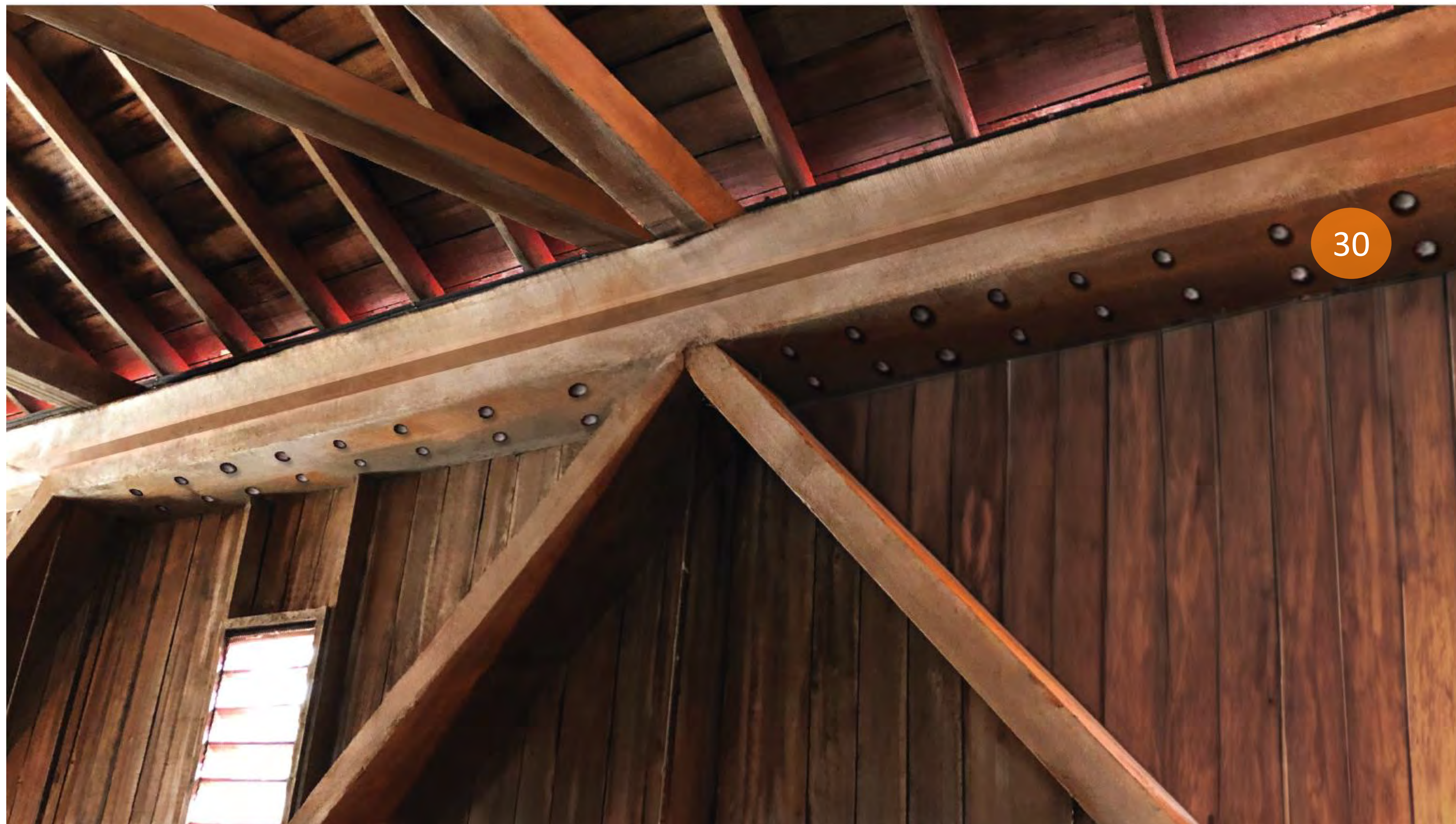
30 Reinforce top chord with lower top chord
