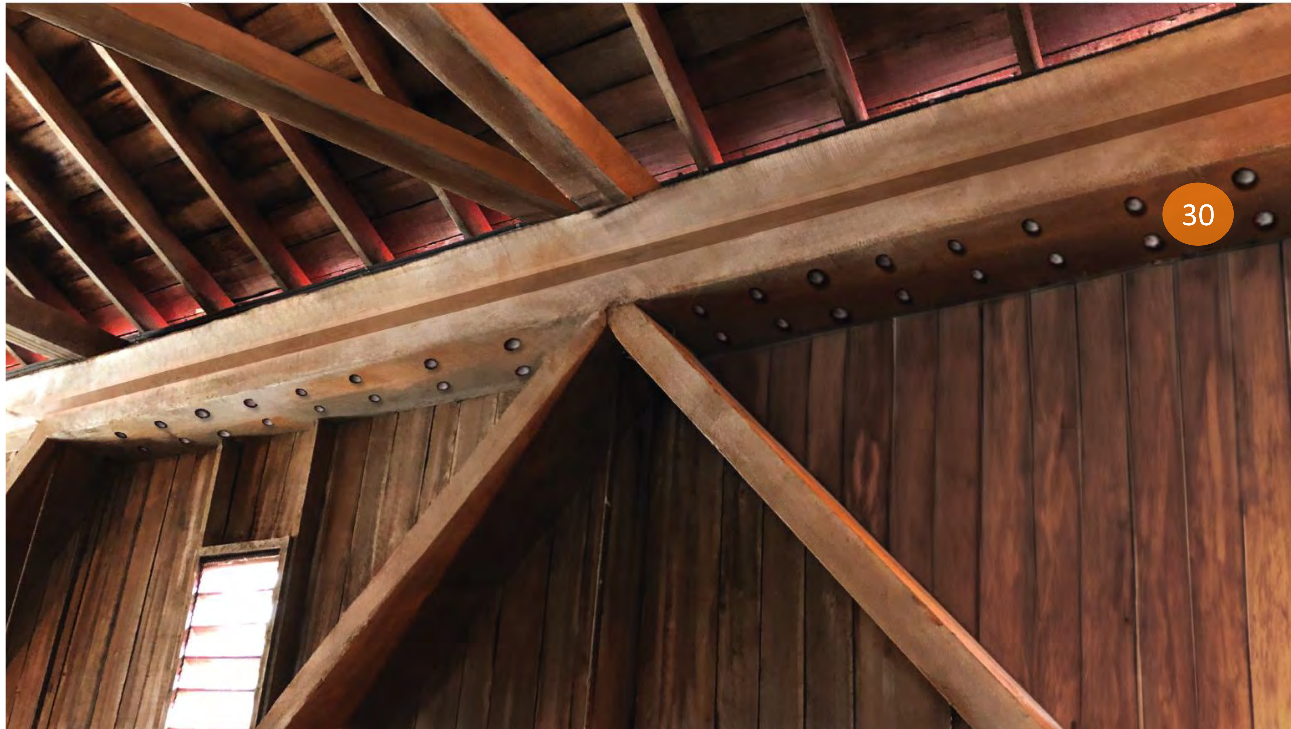
30 Reinforce top chord with lower top chord
