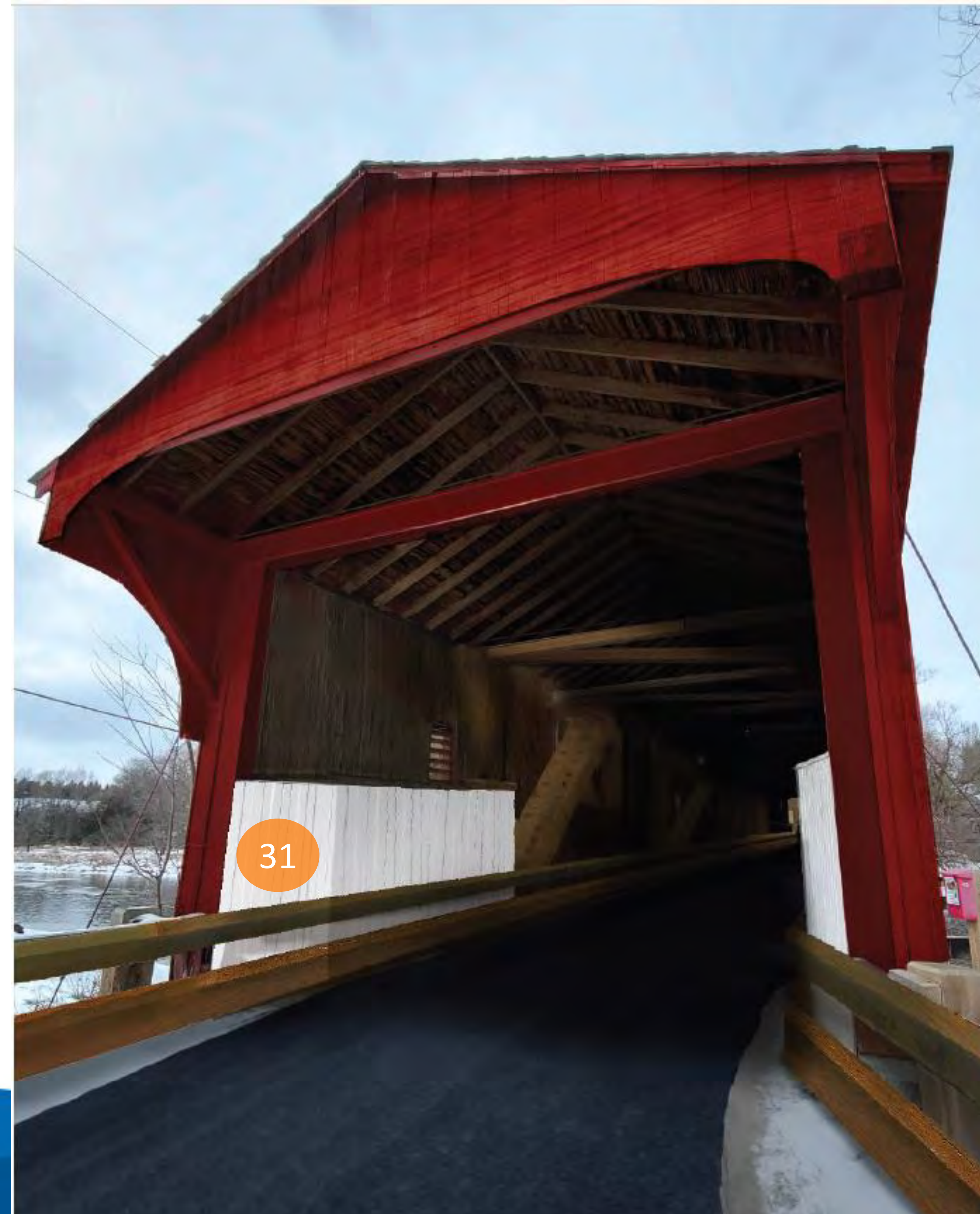
31 Reinstate interior cladding in short sections at each end of the bridge
