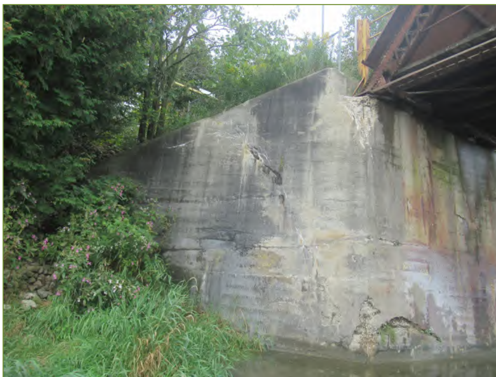
Photo P6 SW Wingwall
