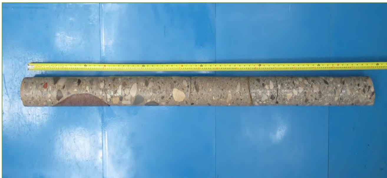
Photo P7 Inside Core C-AB1 (full depth)
