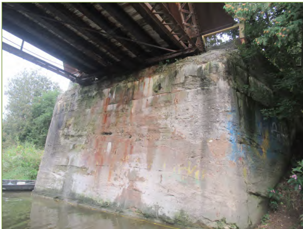
Photo P1 East Abutment
