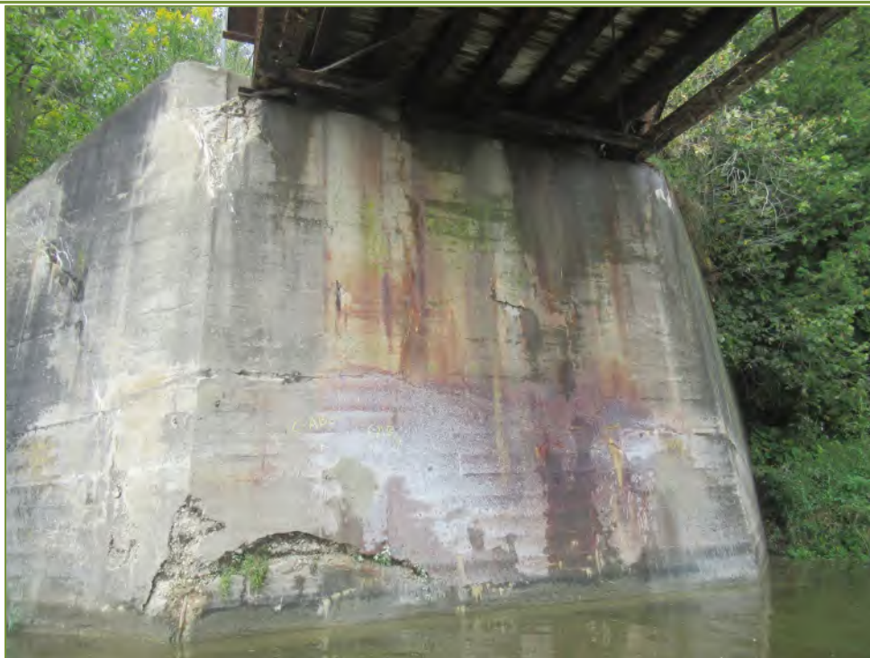
Photo P2 West Abutment
