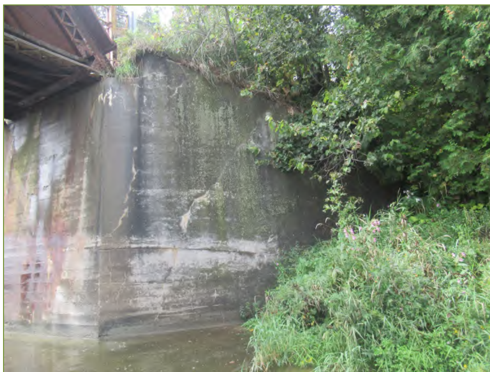
Photo P4 NW Wingwall
