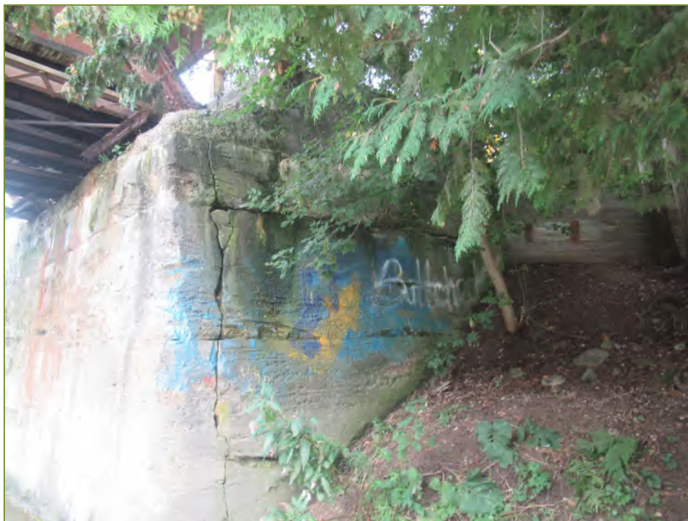
Photo P5 SE Wingwall
